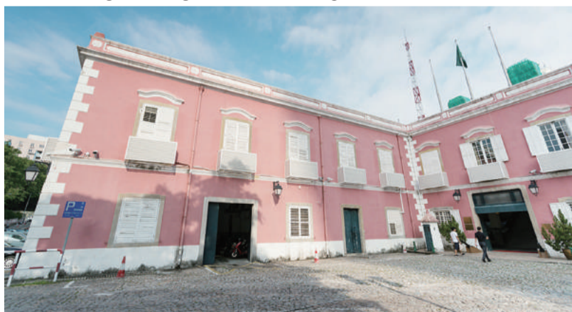
This undated file photo downloaded from the Secretariat for Security (GSS) website last night shows its headquarters in Calçada dos Quartéis.
