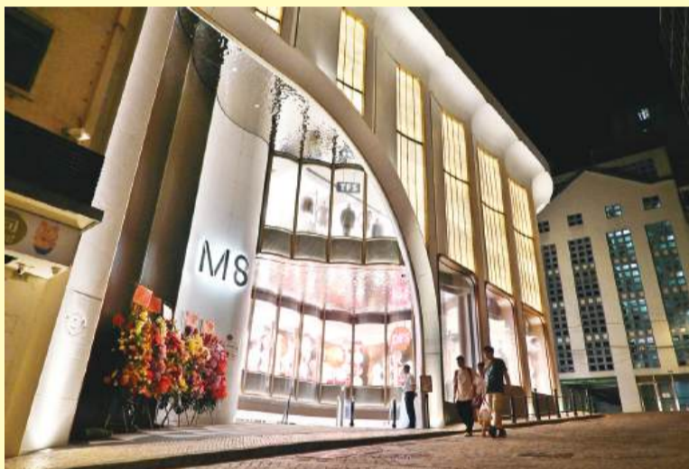
Pedestrians last night walk past M8, which, according to a statement provided by the mall last night, holds the Guinness World Record for the "Largest Curved Stone-Laminated Glass". — Photo: Rui Pastorin
