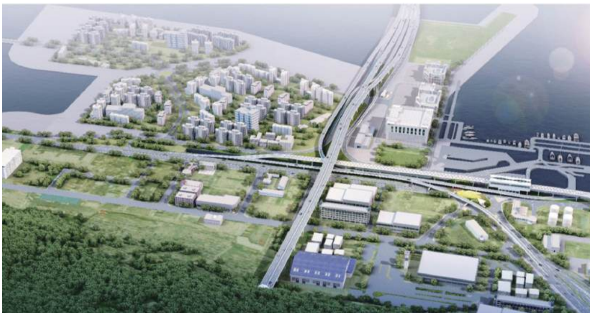
The artist's rendition released by the Public Works Bureau (DSOP) last week show the future flyover linking the future Big Taipa Hill Tunnel's north side with Macau Bridge.
