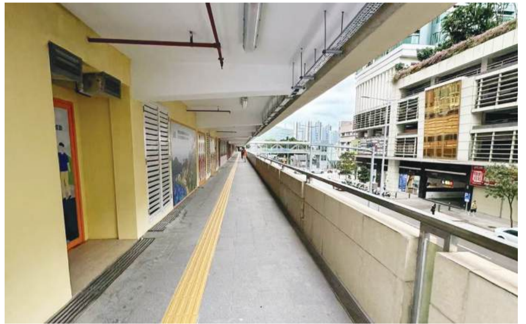
This handout photo released by the Public Works Bureau (DSOP) last week shows a corridor open to members of the public along the podium areas of the Leisure Garden (信愉花園) and San Cheung Seng Garden (新駿成花園) residential estates in Lam Mau Tong.
