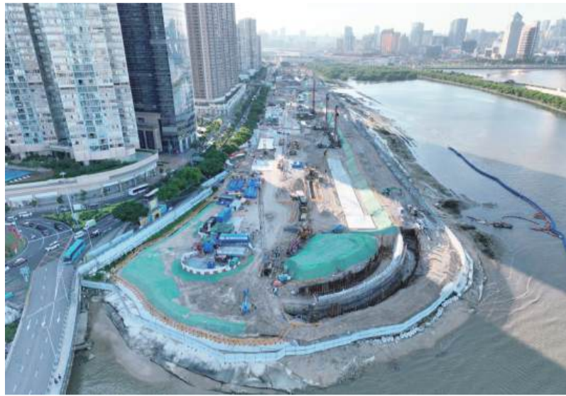
This handout photo downloaded from the Public Works Bureau's (DSOP) website yesterday shows the underwater LRT East Line project including the mudflat reclamation being carried out late last year off the peninsula's northern coast.
