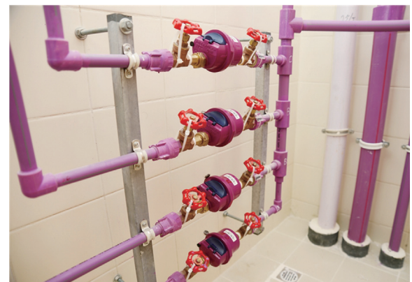
This undated photo downloaded from the Marine and Water Bureau's (DSAMA) website yesterday shows purple pipes in a building used for carrying reclaimed water.
