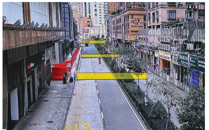
This image shown during yesterday's press conference shows the section of Avenida Dr. Sun Yat Sen in Taipa where the pipework will start on Saturday.
