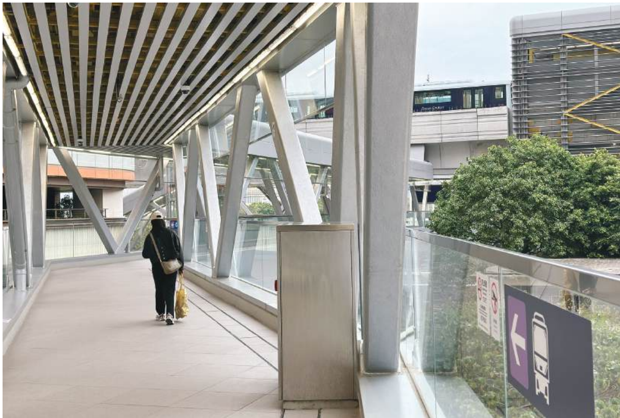
A passenger walks towards the entrance to the LRT Seac Pai Van Line in Coloane yesterday.
