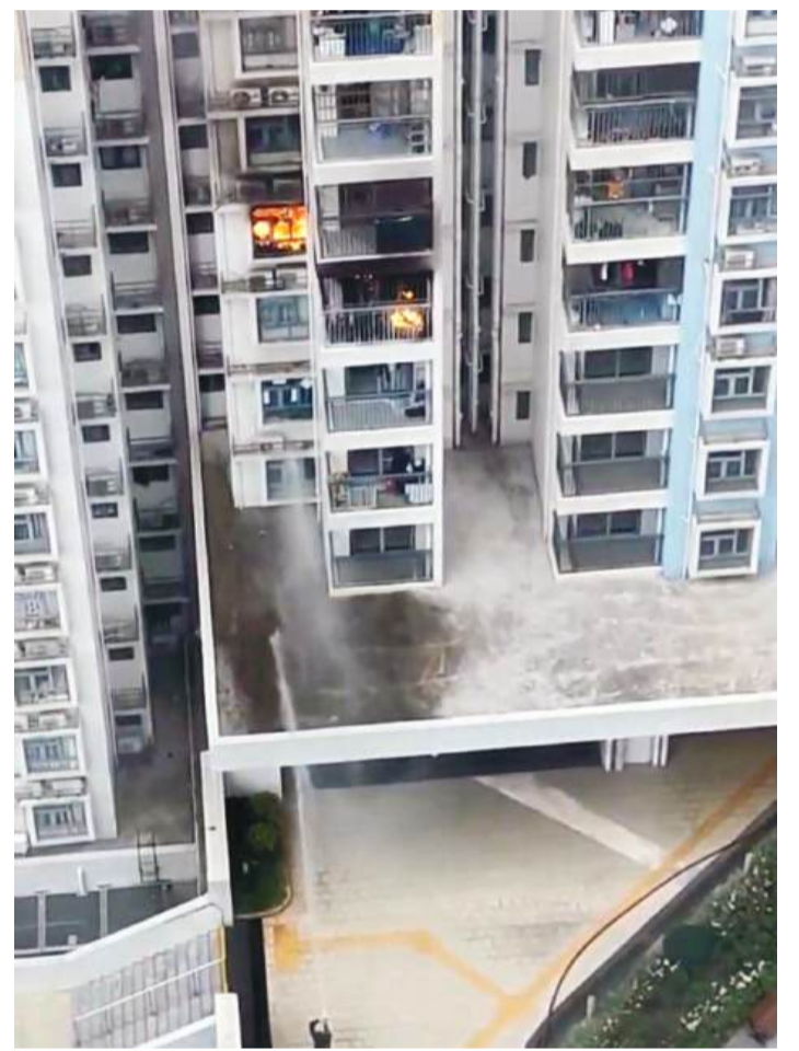
This photo circulating on social media platforms shows yesterday morning's fire in a flat of Block 5 of Lago ("Lake") Building in Taipa.
