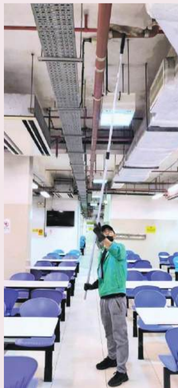
This handout photo provided by the Municipal Affairs Bureau (IAM) shows IAM inspectors at the Iao Hon Municipal Market's cooked food centre cleaning the ceiling pipes of the air-conditioning equipment yesterday.
