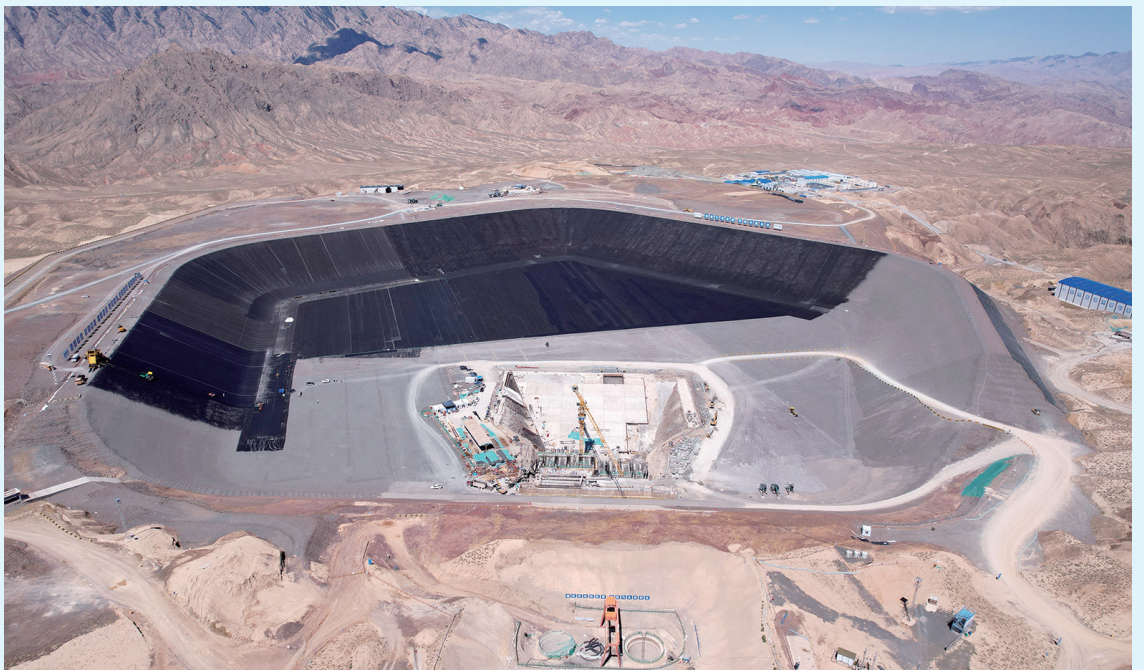
An aerial drone photo shows the construction site of a pumped-storage power station in Zhangye, northwest China's Gansu Province, yesterday. Construction of the power station started in 2022, and all four 350,000-kW reversible pump-turbine units are expected to be fully operational by 2029. A pumped-storage power station is a type of hydroelectric energy storage system that acts like a giant, water-based rechargeable battery. It uses two water reservoirs at different elevations to store and generate electricity on demand.
